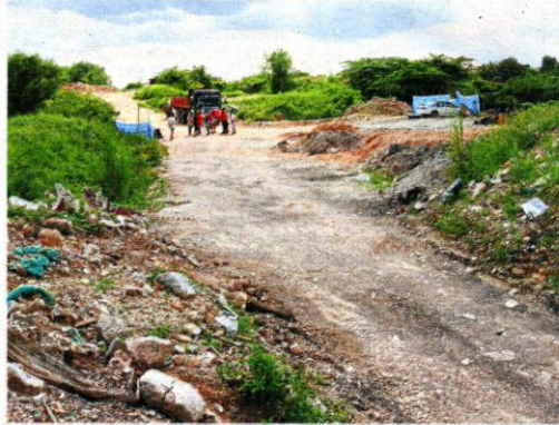
Soil erosion has taken place over the years on a private land in Taman Taynton View.
